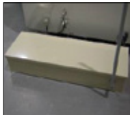
ACC20 Waste Water Trough & Pump
